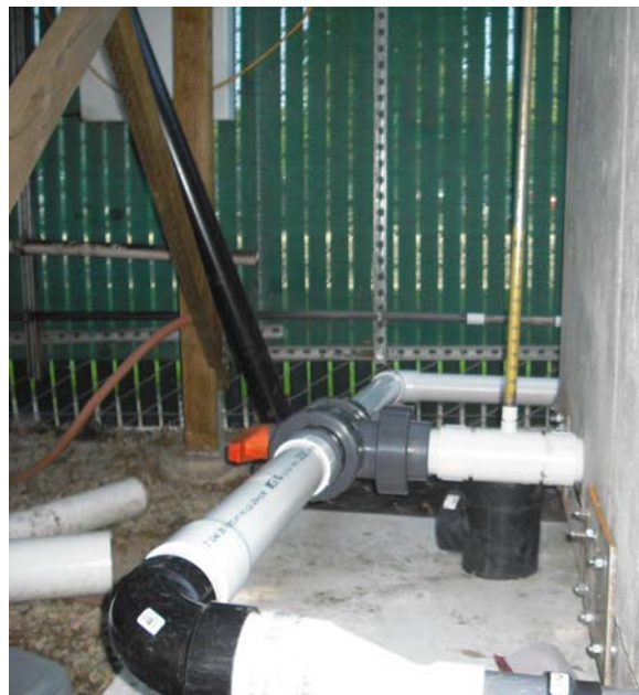
b) 3-inch outlet with 3-inch port ball valve for switching between unrestricted flow in the 3-inch pipe (background) and the 1.5-inch flow meter (foreground)
