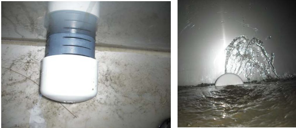
Figure 7 Restrictor Cap and Flow Through Orifice in Restrictor and Exposed Slots in the 3-in Underdrain Pipe
